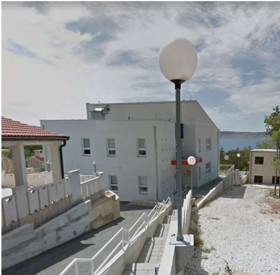
Figure 3-2 Photo of northwest facade
