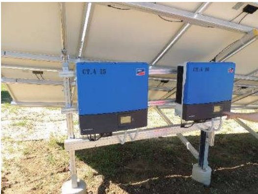
Figure 2-2 Examples of string inverters (left) and centralized high-power inverters (right)
