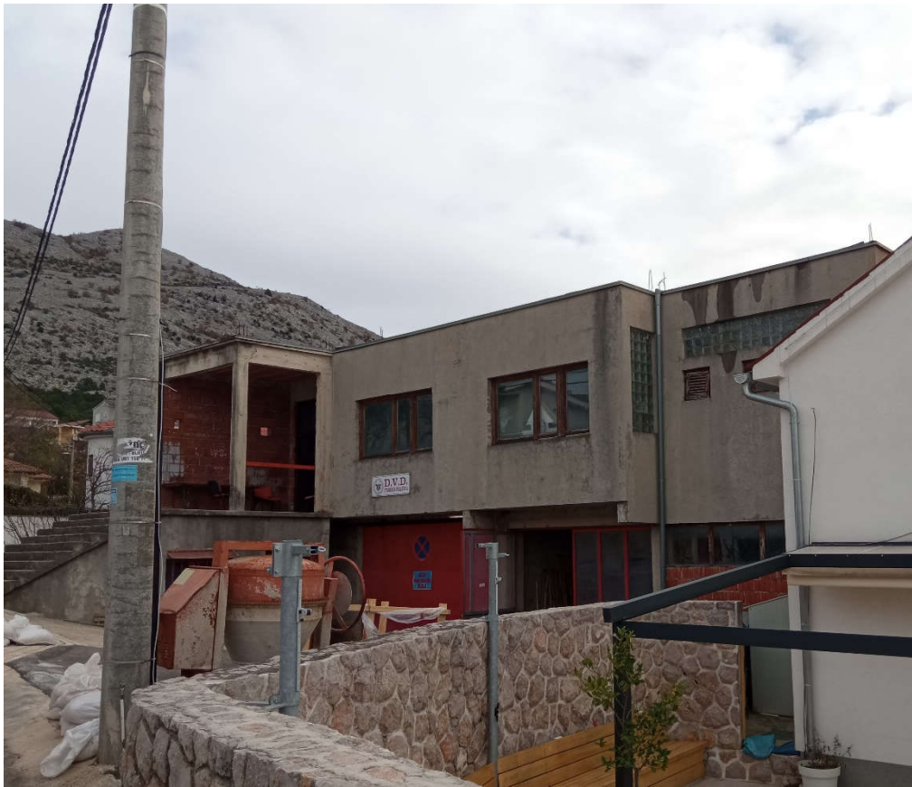
Figure 3-2 Photo of southwest facade
