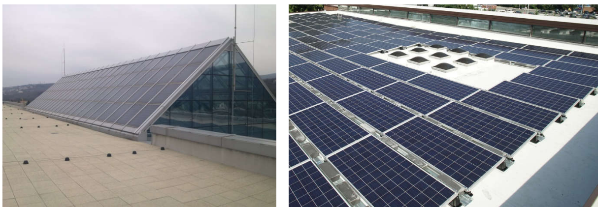
Figure 1-2 An example of a PV system integrated into a building and a PV system on flat roof
