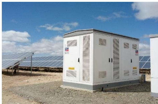
Figure 2-2 Examples of string inverters (left) and centralized high-power inverters (right)
