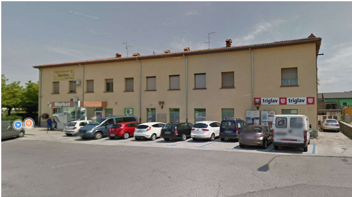
Figure 3-2 Photo of southwest facade
