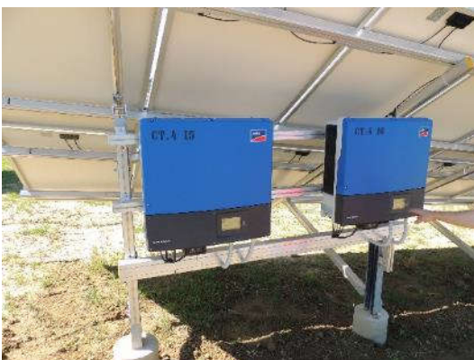
Figure 2-2 Examples of string inverters (left) and centralized high-power inverters (right)
